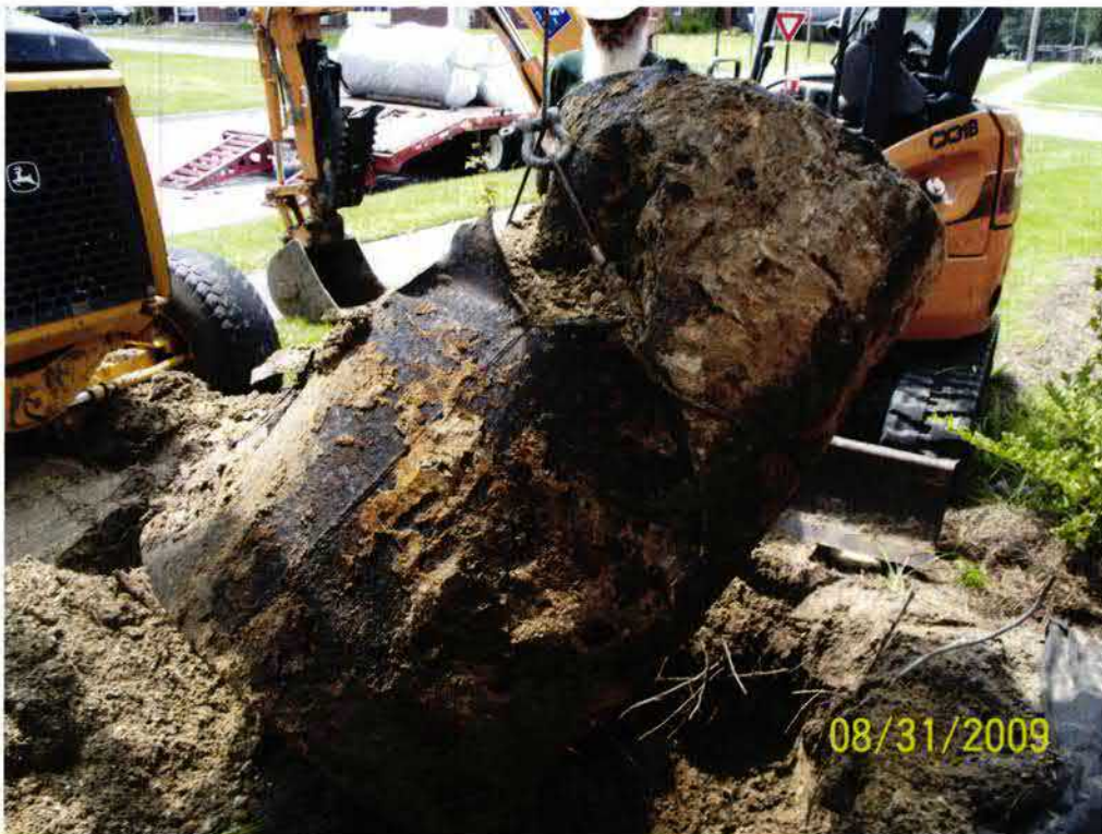
Picture 2: UST 1249Dove removal in progress.
